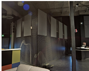
Figure 1: Irregular walls in the main venue
