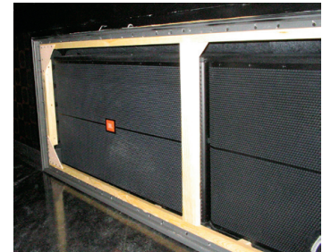
Figure 3: Framed subwoofer enclosure without the fabric installed
