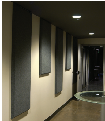
Figure 4: Auralex ProPanels in the backstage area
